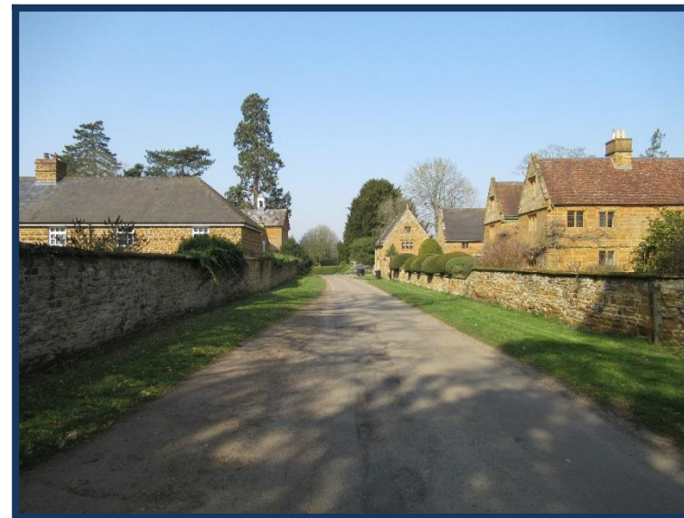
Figure 34: Buildings at the south end of the village, showing the variety of orientations relative to the road
